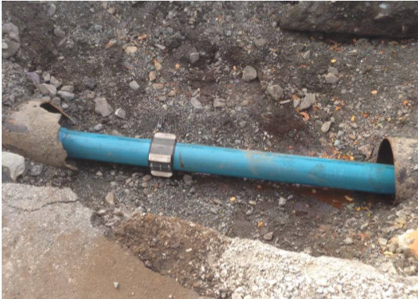
To reduce friction, and to ensure that the TerraBrute CR wouldn't be damaged during the pull, three casing spacers with polyester runners were attached to each length of pipe.
