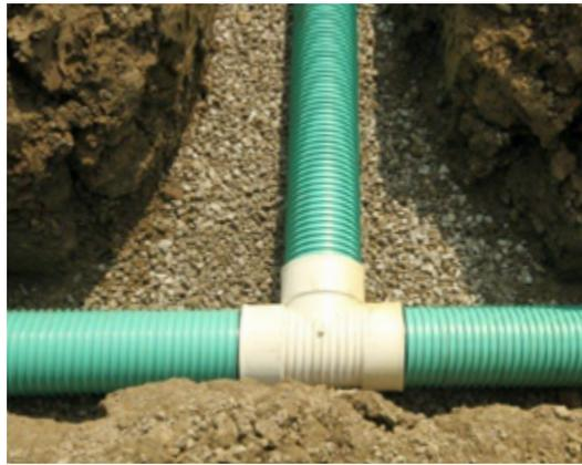
engineers can ensure leak-free joints that are watertight and air-tight by simply **specifying sewer pipe and fittings from a single manufacturer with joints that are third-party certified to a hydrostatic pressure of 50 psi and by specifying low-pressure air testing in the field to an air pressure of 5 psi per CSA B182.11.**
